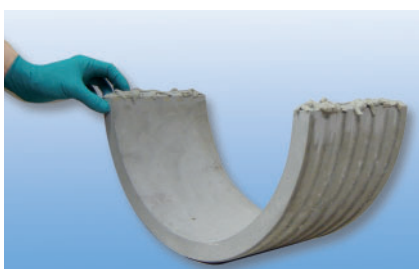
Apply filler thickly to both half casings and press in spacer (included in the delivery) (distance to half casings 5 mm).
