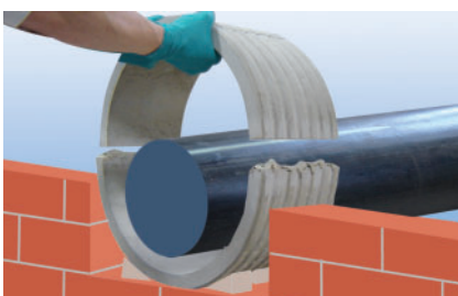
Connect half casings for fit until both halves rest on spacers.
